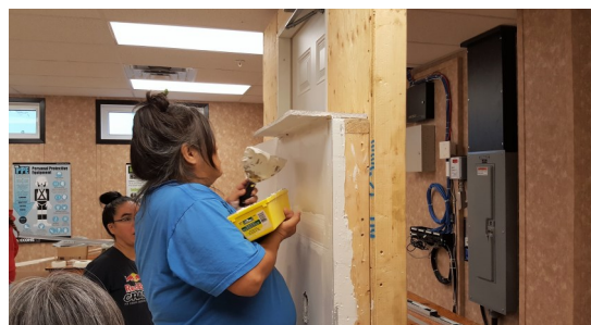
Denita Bird applies drywall compound to a gypsum board
