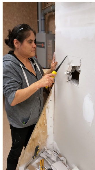
Elizabeth Gee measures surface for drywall
